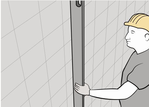
Check planarity of the existing substrate
