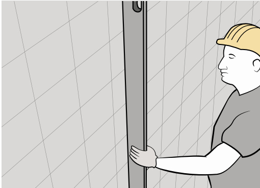
Check planarity of the existing substrate
