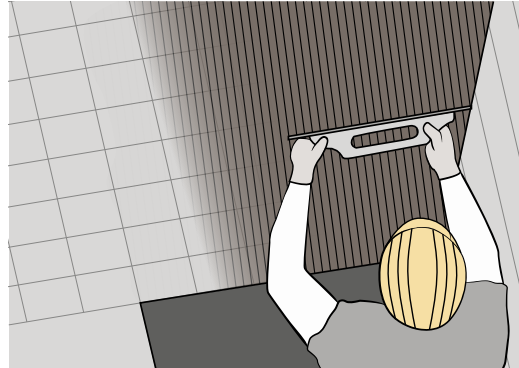
Spread adhesive on the existing substrate
