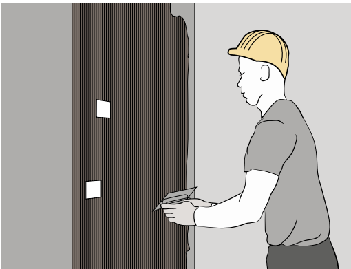
Spread adhesive on plaster
